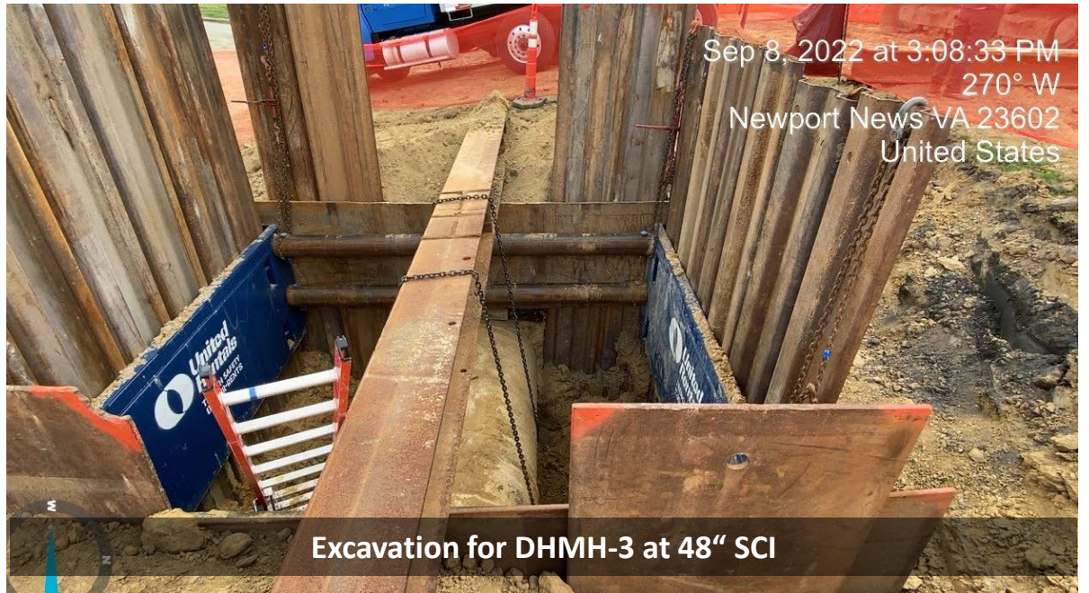
Excavation for MH's 3 & 4
